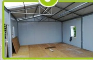
Install the floor and roof
