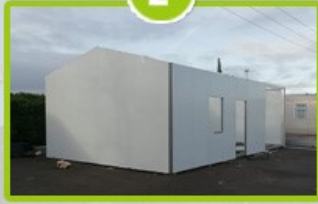
Install the sandwich walls
