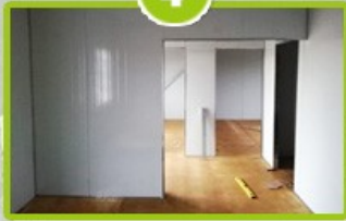
Install the partition walls
