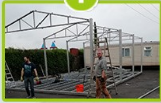
Install the steel structure
