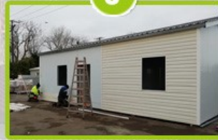
Install the cladding wall
